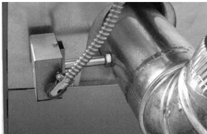
Figure 4 – Position de montage acceptable 2
