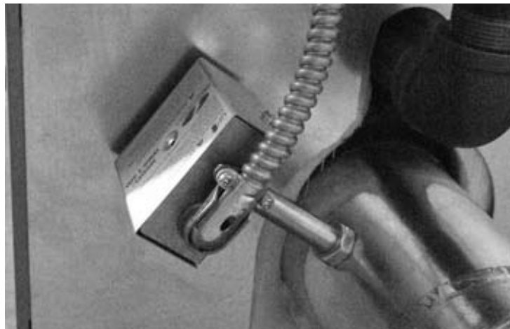
Figure 3 – Position de montage acceptable 1
