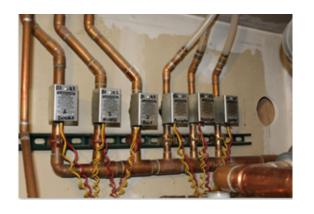
Kyle jumped at the opportunity to upgrade the existing 16 year old Cast Iron boiler. The unit had an input of 396 MBH and 6 zones, the bottom shop floor heating 5250 sq. ft. (with in-floor heat) and the upper two floors heating 1550 sq. ft. with standard fin-tube. A 40 gallon gas fired water heater tried to keep up but all too often was unable to meet the heavy demands.
