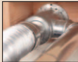
Flexible Vent Pipe
